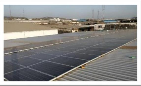
Solar rooftops installed at both of our warehouses with a combined capacity of 240 KW. The solar rooftops generated 221 MWh of power.
